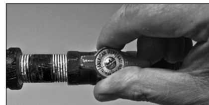
Figure 42 - Gas valve in "on" position.
