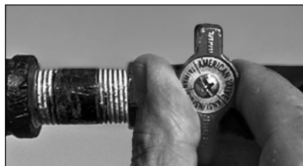
Figure 40 - Gas valve in "off" position
