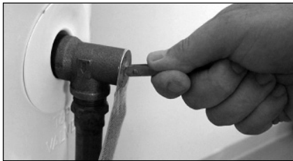
Figure 37 - T&P Relief Valve.
