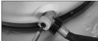
Figure 34 - Draining the water heater.
