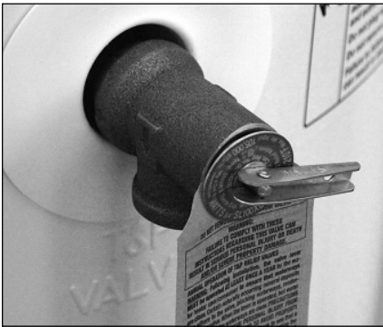
Figure 22 - Temperature and Pressure Relief Valve
