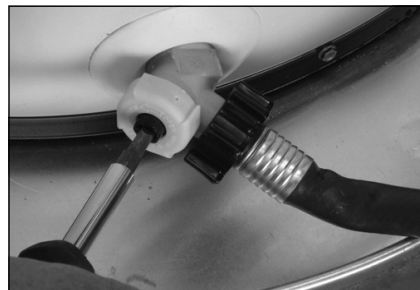
Figure 19 - Draining the old water heater.
